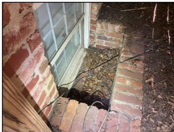
12. Less than 6 inches below window
