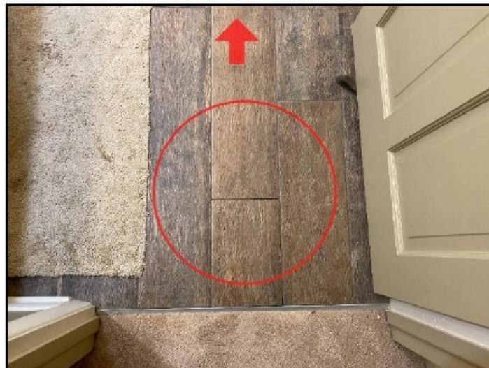
69. Grout missing
